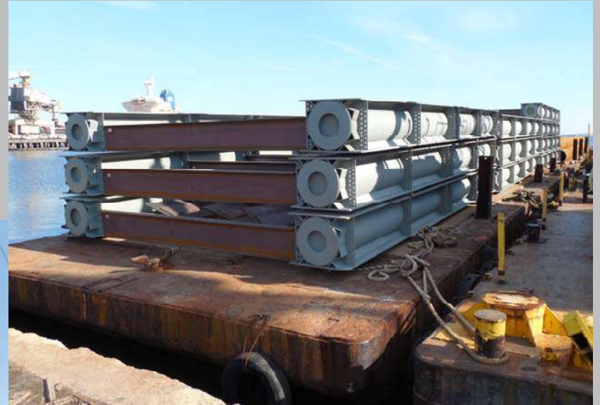
Barge loading 70% complete
