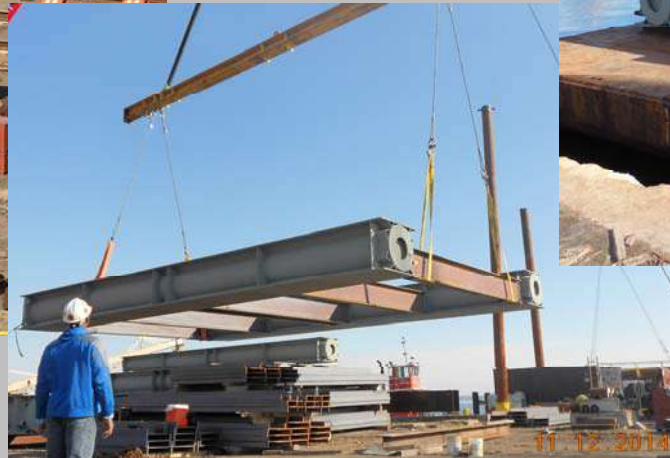
Span by span loaded to barge
