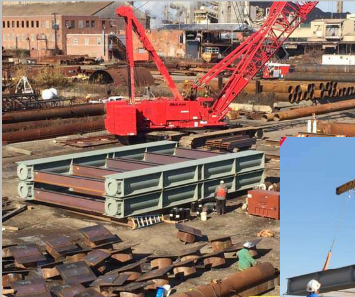
Frame style trestle in 40 ft. sections
